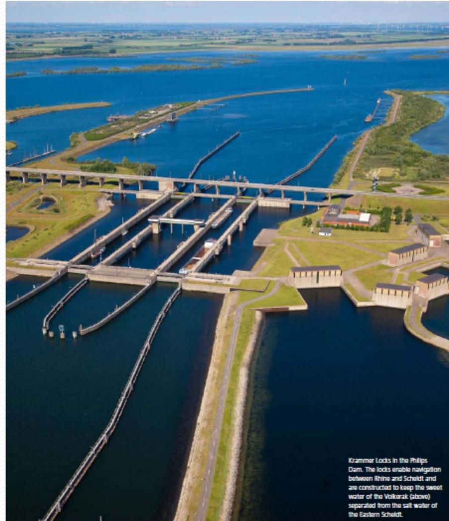
Krammer Locks in the Philips Dam. The locks enable navigation between Rhine and Scheldt and are constructed to keep the sweet water of the Volkerak (above) separated from the salt water of the Eastern Scheldt.
